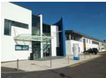
Crosshouse Maternity Hospital, UK
